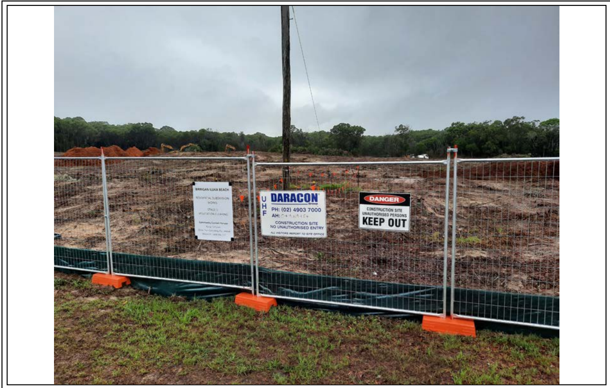
Photo 1: Wood chip operation in progress. Looking from Micalo + Elizabeth Street intersection to the project site.
