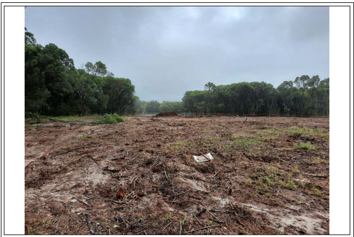
Photo 6: From northern Stage 1 clearing boundary looking south towards existing bushfire trail fence behind stockpile and Lot 1 (Park C) partly behind fence + part red flag demarcation.
