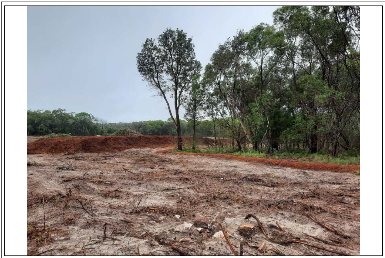
Photo 2: Wood chip stockpile north of Lot 1 Park C + F. Wood chip mulch berm to Lot 1 perimeter.
