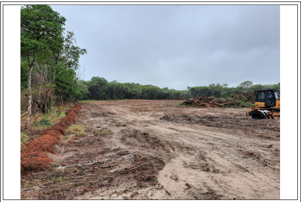
Photo 4: Wood chip / mulch berm to edge of vegetation clearing along north / eastern internal boundary taken from existing access track.
