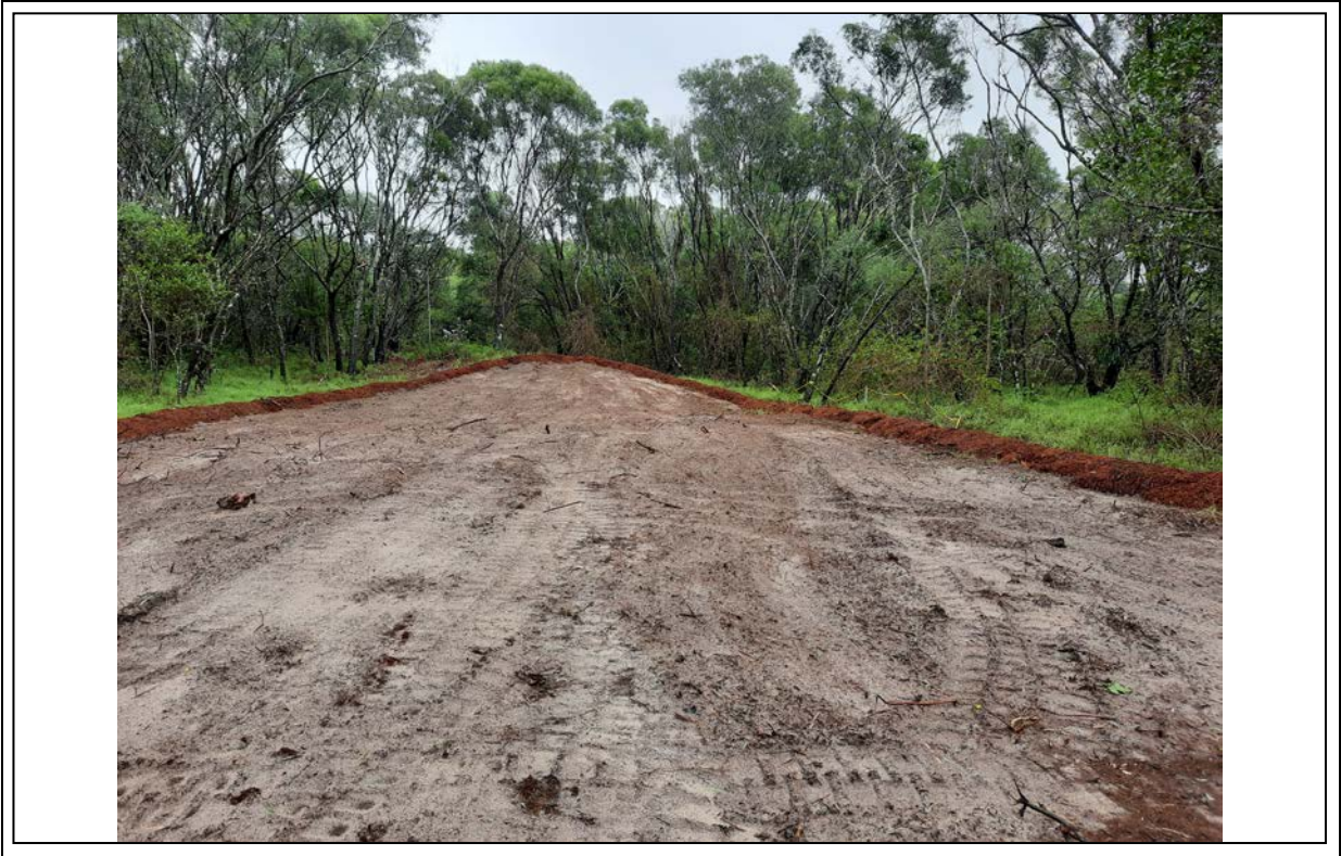
Photo 7: Wood chip / mulch berm to perimeter of construction compound area off Lot 7020 + Hickey Street.
