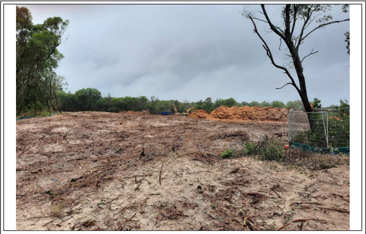
Photo 3: Excavators feeding wood chip grinder on western portion of Stage 1 looking from Elizabeth Street future emergency access position.
