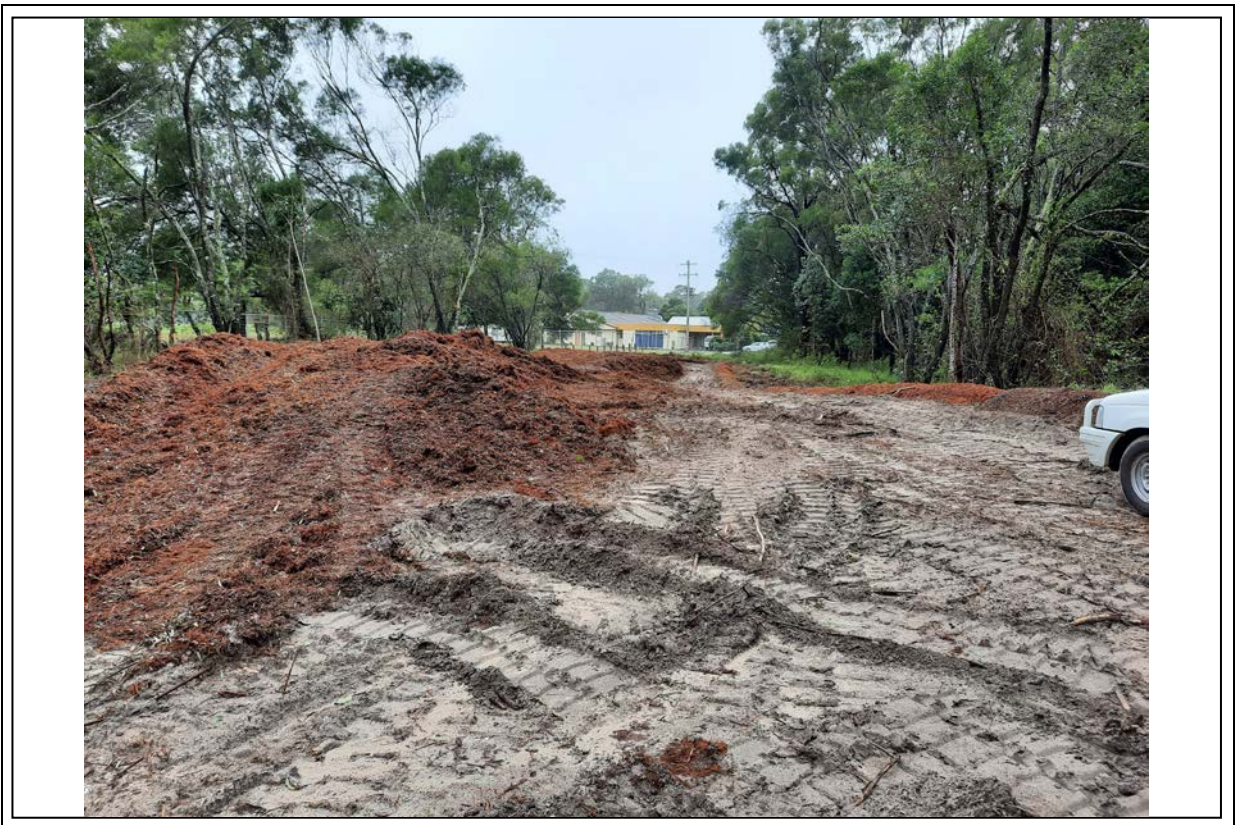
Photo 8: Wood chip / mulch stockpile + berm to perimeter access to Hickey Street looking from site towards Iluka Golf Club.
